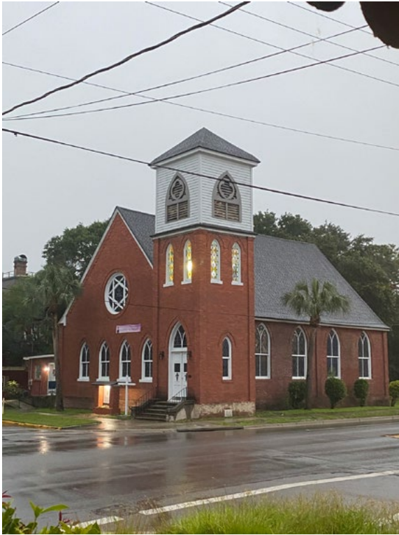
Trinity United Methodist Church, c.1891, in Fernandina Beach's Downtown Historic District at 715 Ash Street. Trinity is associated with the African American community in Fernandina and the building construction was largely funded by freedmen and women. Credit: Adrienne Burke
