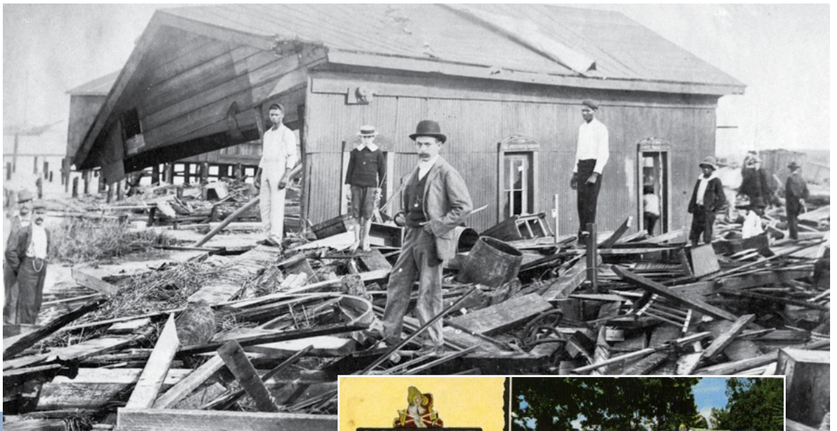
Right: Downtown Fernandina after September hurricane, 1898. Storms have historically impacted Nassau County and continue to remain a threat to historic and cultural resources. Credit: Library of Congress
